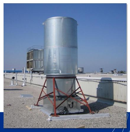
Mndustrial process centrifugal fan intake & discharge
